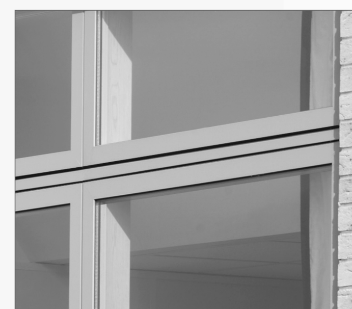
Ventilation position. The striking plate allows a 5mm night ventilation opening for all espagnolette handles.
